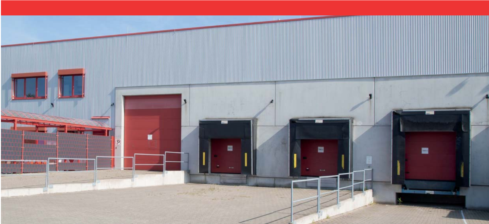
Exterior lights – exterior application – entrance area with FL2N-LED
